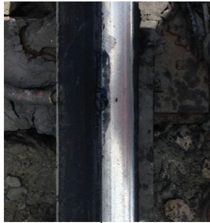
TOR Armor filling holes in rail head.
